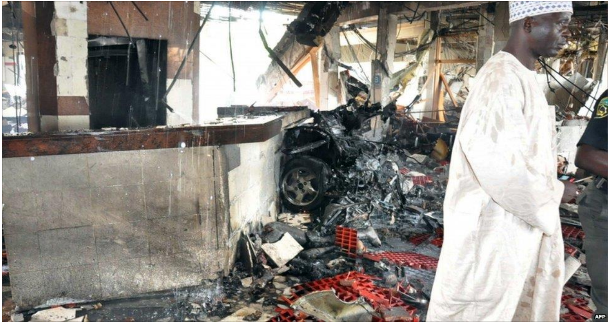
Figure 2 United Nations photograph of the car bomb. Notice how the block counter wall remained in place? While the people in the room were killed by the concussion and explosion, this is an excellent example of how reinforced concrete can stop a car bomb.
